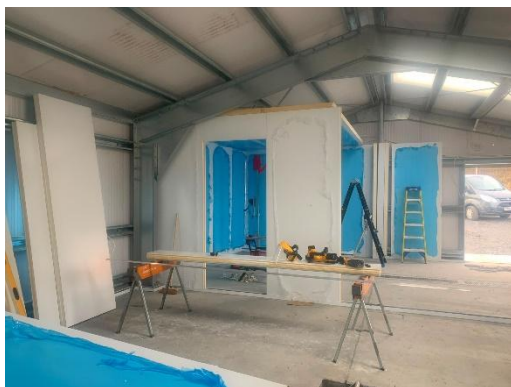
During construction of Wild Jura Venison AGHE
